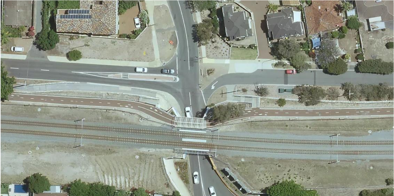
Figure 7-38 Stirling Road / Claremont Crescent – existing intersection
