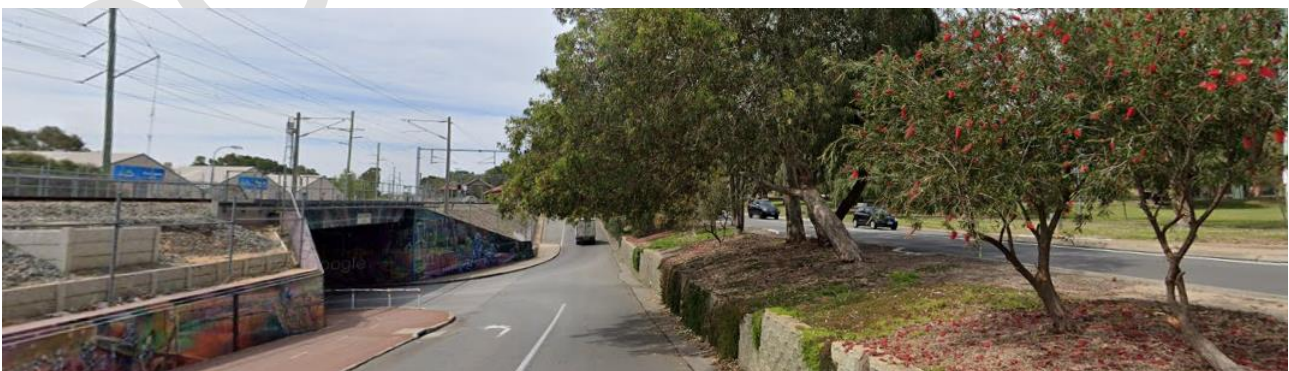
Figure 7-32 Shenton Road subway – level difference
