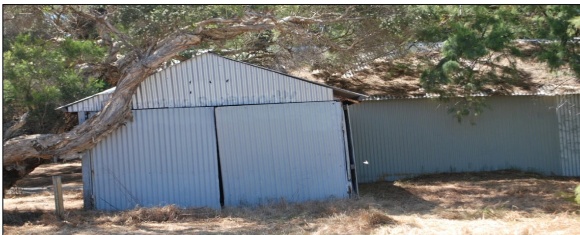
Figure 3.3: Storage shed with overhanging tree
