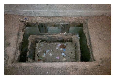
Figure 5: Stormwater drain insert to collect sediment
