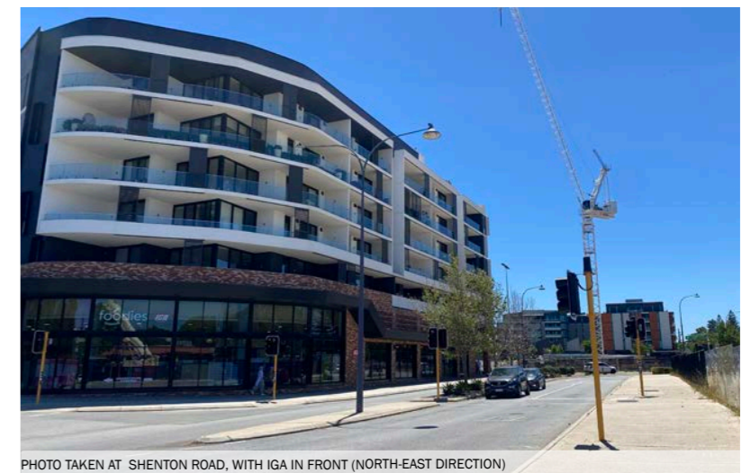
PHOTO TAKEN AT SHENTON ROAD, WITH IGA IN FRONT (NORTH-EAST DIRECTION)
