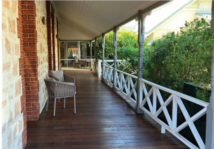
4 Verandah Around Homestead
