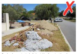
Sand and concrete stockpiled outside of construction site.
