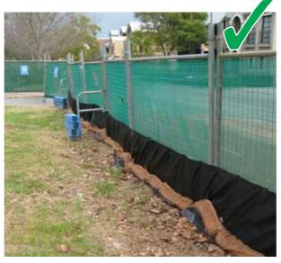
Secure the geotextile material to the perimeter fence to a minimum height of 600 mm.
