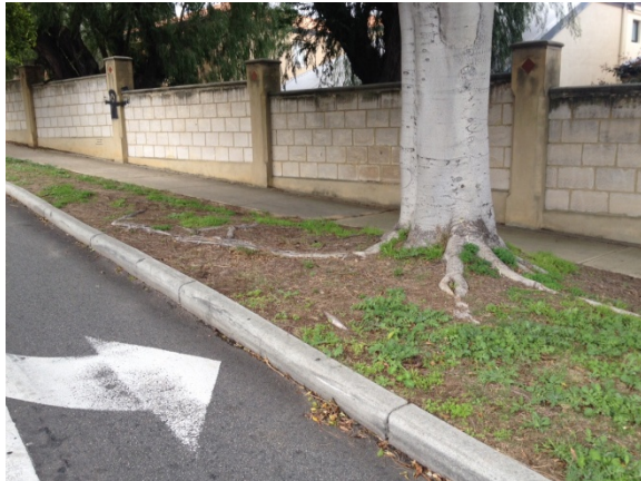
Ficus Tree "A" - Image 3 and 4 - Lifting of curb causing separation from bitumen, proximity to traffic lights and highway
