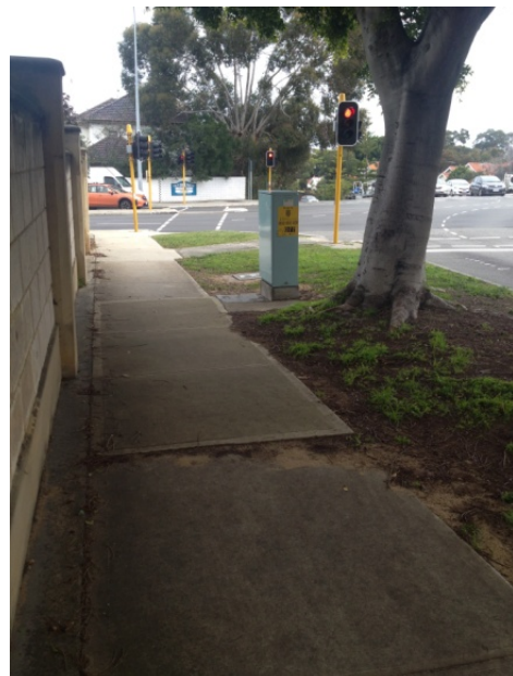
Ficus Tree "A" - Image 1 and 2 - Damage to MRWA traffic control infrastructure and footpath heave
